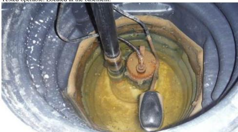
Pump was activated at the time of inspection and found to be in good working condition. We suggest you verify proper operation on an annual basis. Failing pumps can cause basement seepage during heavy rains. A good commercial pump should have an average life expectancy from 7-10 yrs.
