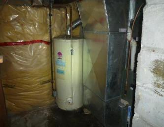
2111.Maintenanc<br/>eReview. Leaks observed, suggest review by qualified plumber<br/>for repairs/replacement as necessary.
