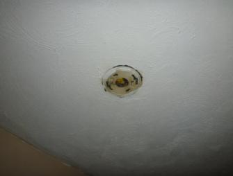
1809. Electrical Comments Review. The electrical system is an older non-grounded 2wire system. This was common practice when this house was built. Due to safety concerns, it is suggested client consider upgrading to a new 3-wire grounded system or GFCI protection to enhance electrical safety. A review by a licensed electrician prior to closing for upgrading the electrical system is suggested.
