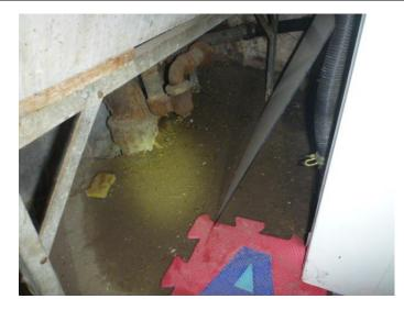
Although no leakage was detected, there appears to be a nonstandard repair at the drain line at basement, which is temporary in nature, permanent repairs are needed.
