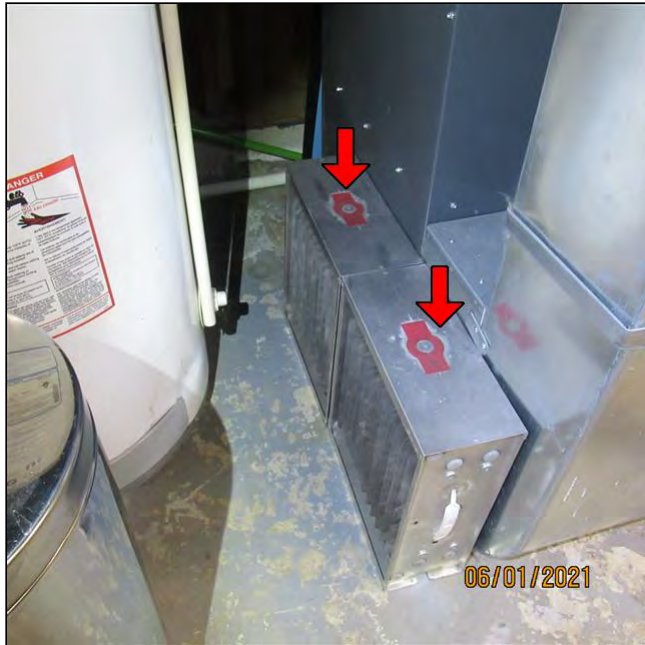
12.5 Item 3(Picture) Electric filter elements
