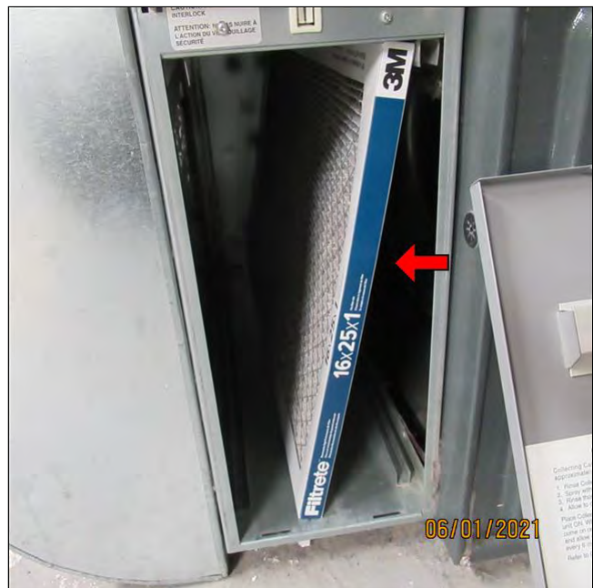
12.5 Item 2(Picture) Poorly fitting disposable filter media
