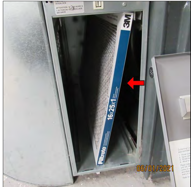
12.5 Item 2(Picture) Poorly fitting disposable filter media
