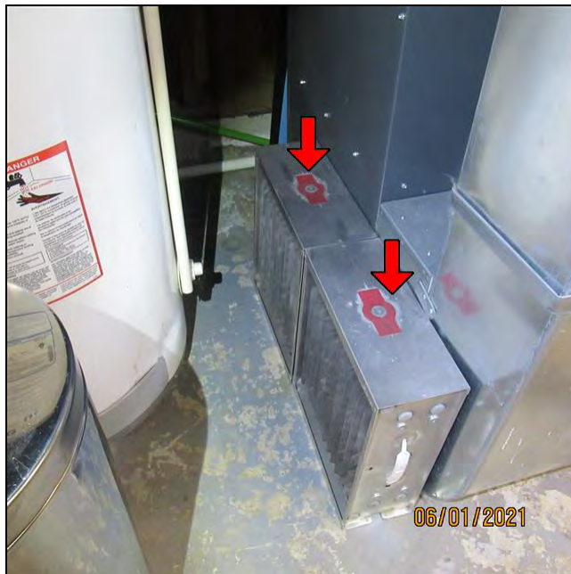
12.5 Item 3(Picture) Electric filter elements
