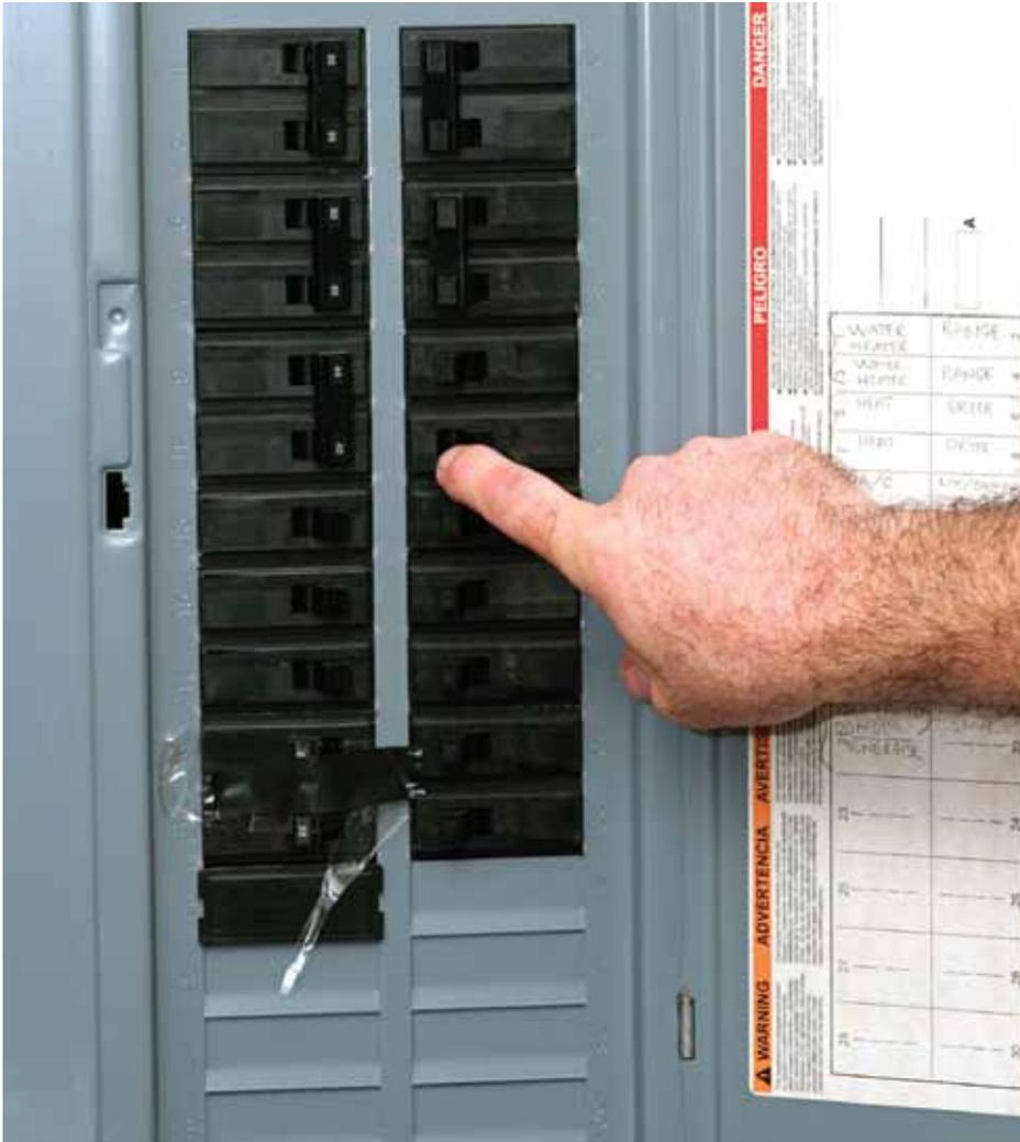
The electrical service provided to a home is measured in amps, which is a measure of the “flow rate” of electricity through a wire. Today’s average home is constructed with electrical service of 100 amps, which means that the large main wires entering the home can safely handle 100 amps of current before there is a risk of overheating. Some homes,
