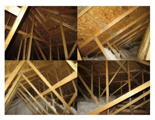
1910. Sheathing Serviceable. Waferboard/OSB.
